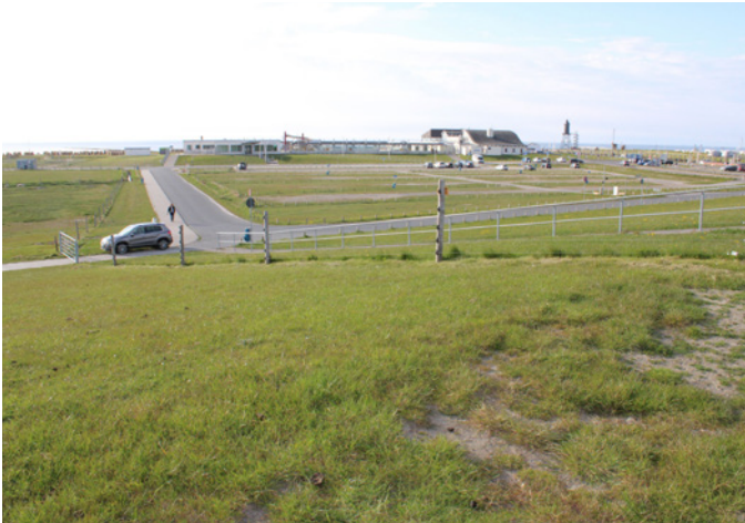
Fig. 9. Wolf-deterrent permanent electric fence on a sea dyke next to tourism infrastructure (Photo: Peter Schütte).
