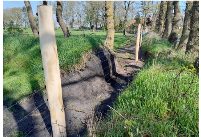
Fig. 10. A high electric fence (with wires at 20, 40, 60, 80, 105 and 130 cm plus polywire to increase visibility at 155 and 180 cm above the ground) to deter wolves from using the adjacent hedge bank to jump over (Photo: Peter Schütte).
