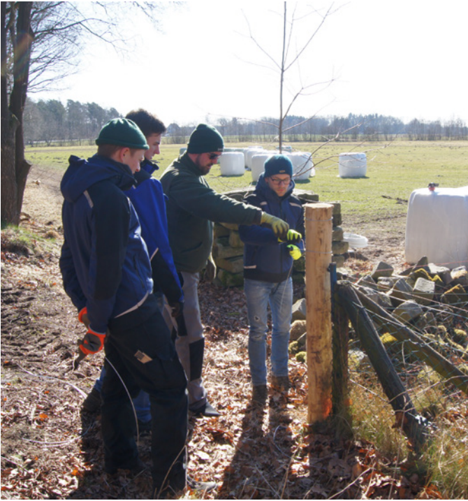
Fig. 5. Project volunteers being trained in fence construction (Photo: Peter Schütte).
