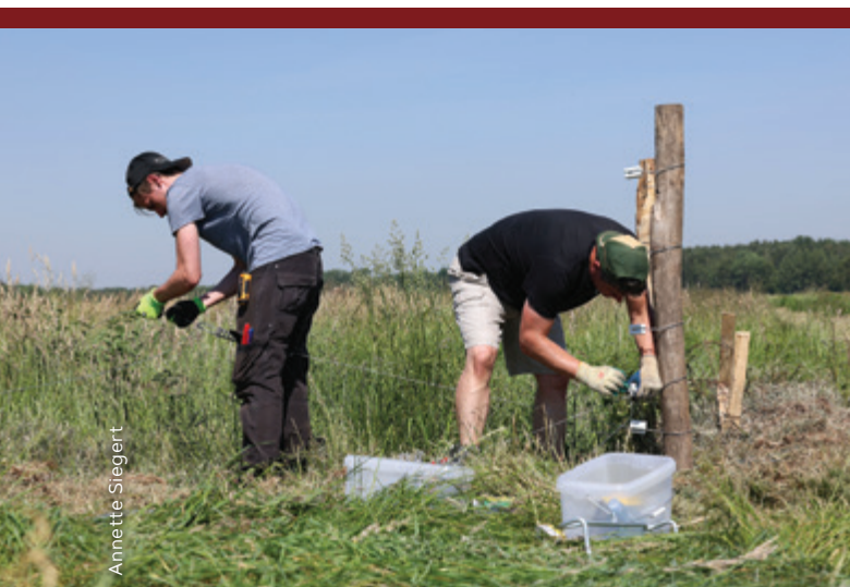
Volunteers constructing a wolf-deterrent permanent electric fence
